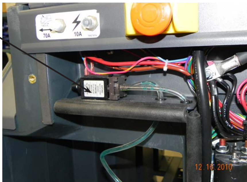
Detergent (Chemical) Pump
